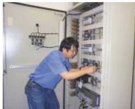
Maintenance à Hong Kong PSD maintenance in Hong Kong Metro
