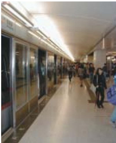
Portes palières Hong Kong Hong Kong Platform Screen Doors
