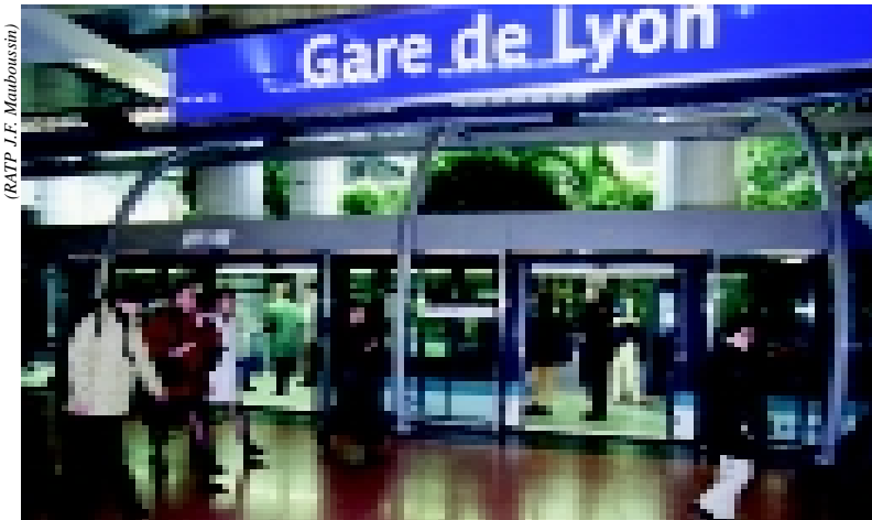
Portes palières Faiveley, station Gare de Lyon de la ligne 14 (RATP). Faiveley platform screen doors, gare de Lyon station on Paris line 14 (RATP).
